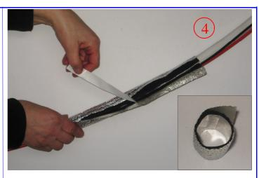
Verify that the closure of the sleeve results in the overlap of the two strips of black fiber and that there is continuity along the diameter of the insulation. Remove the external liner.
