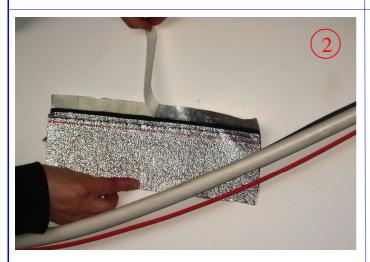
Characteristic of this sleeve is that there is a double bonding interior - exterior. You will have to remove the liner from the internal adhesive (side lines).
